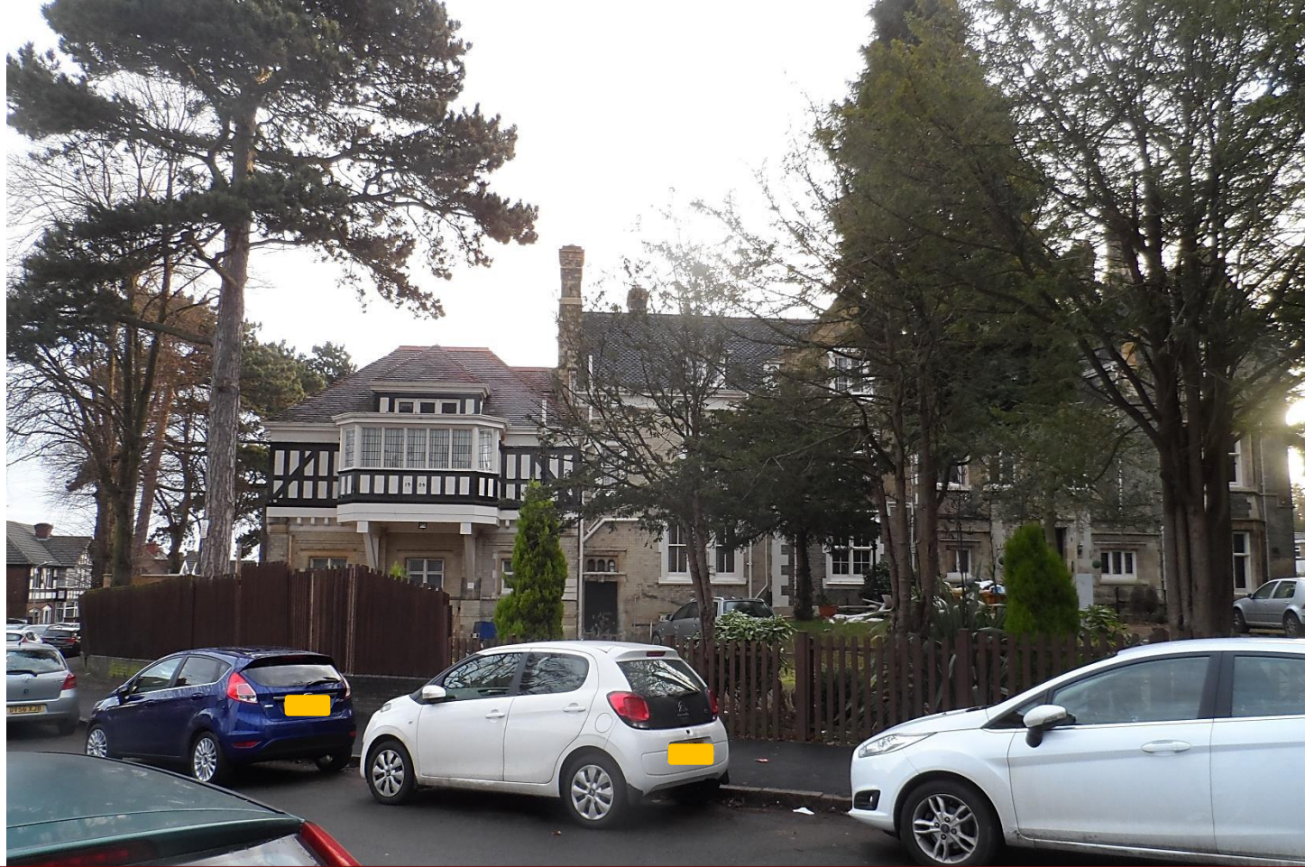
Front of building
